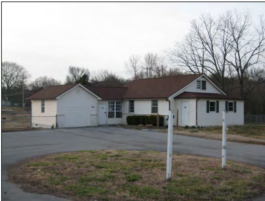
SOUTHEAST FRONT VIEW OF EXISTING BUILDING
