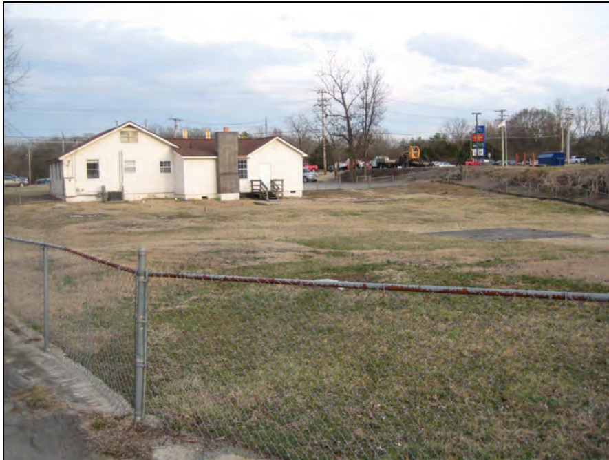
SOUTHEAST VIEW OF SUBJECT SITE AND LOCATION OF SINKHOLE
