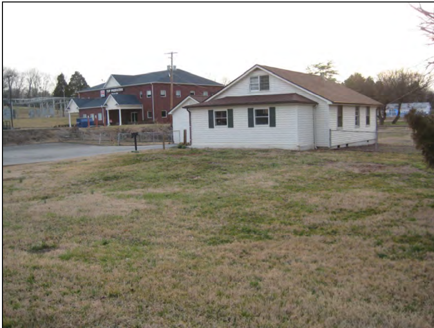
SOUTHWEST VIEW OF SUBJECT SITE
