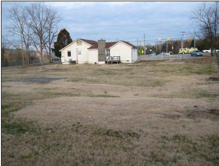
NORTHEAST VIEW OF SUBJECT SITE AND LOCATION OF SINKHOLE
