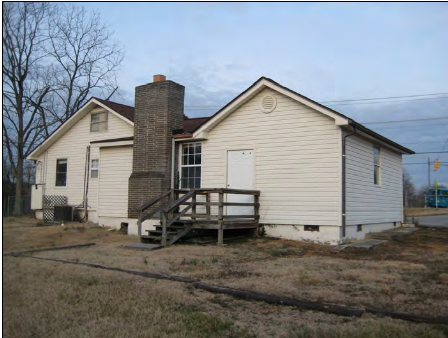
SOUTHWEST REAR VIEW OF EXISTING BUILDING
